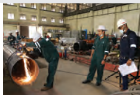
PIPE FABRICATION WORKS
